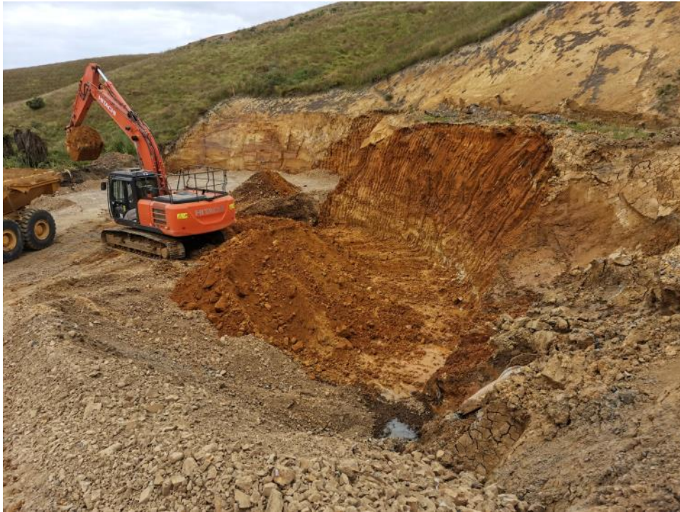
12D topsoil horizon stripping:
