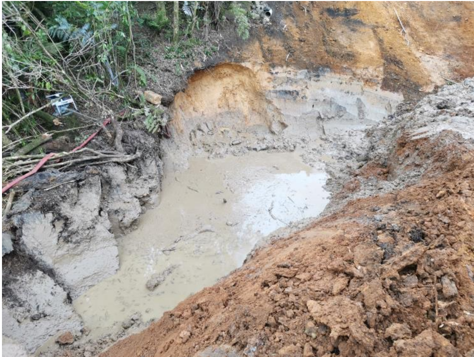
Damaged underfill drain in REB2:
